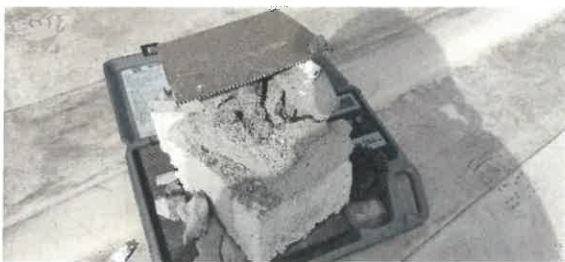
Photo #17 General overview of the make-up of core 'F'.
