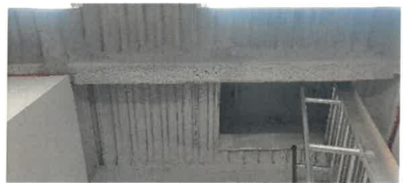
Photo #4 Underside of the roof decking.
