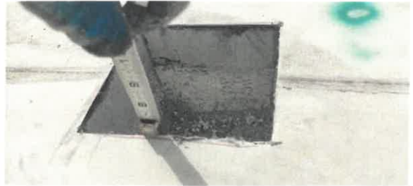
Photo #14 Close-up view of core 'D'.
