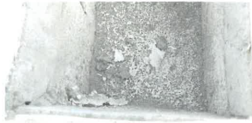
Photo #20 Close-up view of core 'G'.
