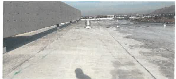
Photo #2 Overview of the north section of the building.
