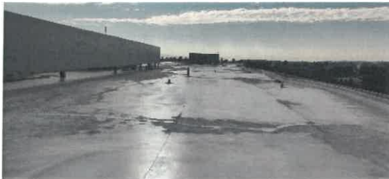
Photo #1 Overview of the south section of the building.
