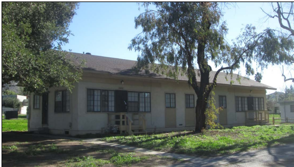
Figure 15: Two-bedroom duplex unit on Utah Street.
