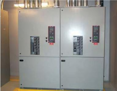
The emergency power system will be capable of picking up their rated capacity in one step and provide a transition time for the emergency systems within ten (10) seconds for the Life Safety Loads and within (60) seconds for the legally required and optional standby loads from failure of the normal power source.
