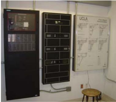
The control panel will receive all alarms from peripheral devices and remote data gathering panels, initiate a pre-recorded voice message throughout the facility, and indicate alarm on the floor of incident and the floor above.
