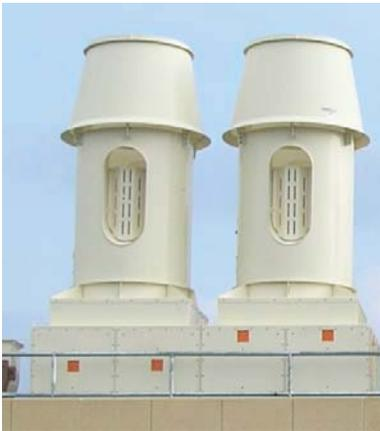
All exhausts will discharge a safe distance above the roof to prevent recirculation through proper dispersion of the air stream into the atmosphere. Discharge stacks will be designed to release the exhaust air at a minimum level higher than any human working on the roof and at a sufficiently high velocity to enable the exhaust air to disperse. The final height, location and discharge velocities will be in accordance with the Wind Consultant’s recommendations.
