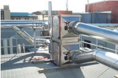
HEPA /Carbon filters will be provided. The system will be on emergency power and equipped with 100% redundant fan and filter bank.
