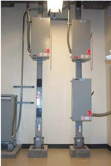
Lighting panel(s) will be provided on each floor that are fed from the busway plug-in circuit breaker(s) which will be equipped with ground fault protection.
