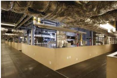
Ductwork from the fume hoods to the linear exhaust valves will be stainless steel.
