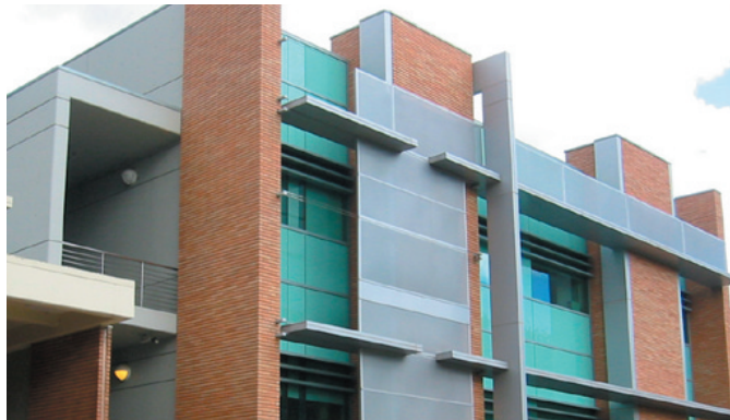
Material palette from the Chemical Science Building
