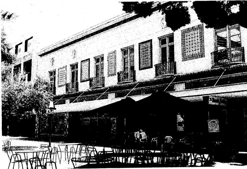
Rouse Building, West Front, 2002
