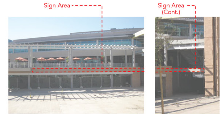
Existing Condition (Location: sC.1)
