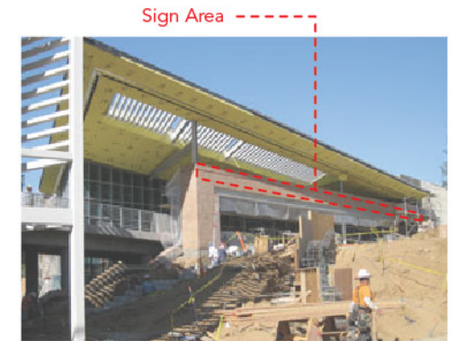
Existing Condition (Location: sC.2)
