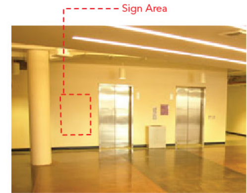
Existing Condition (Location: wB.1)
