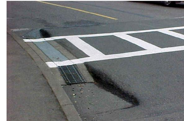
Figure 5.25: Example of a Raised Crosswalk
