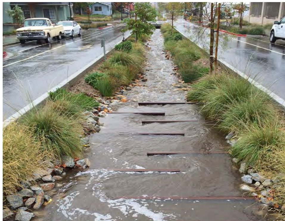
Stormwater facility in roadway median, Paso Robles, CA
