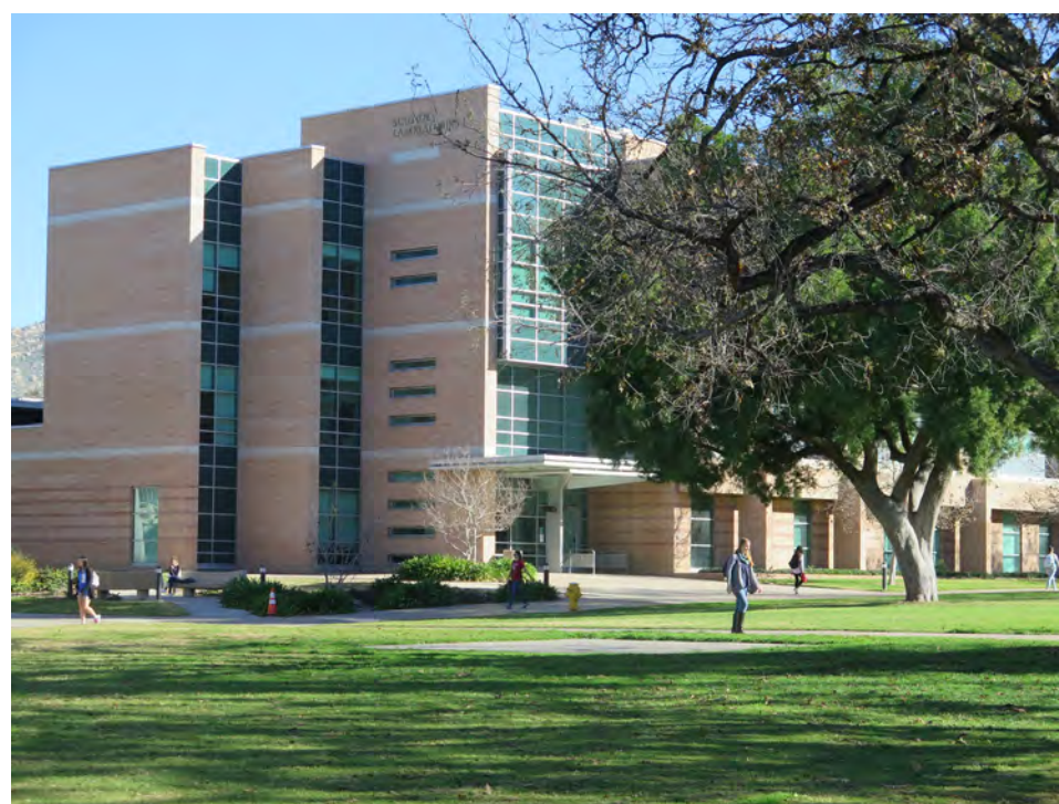
Pierce Hall opens to the Carillon Mall
