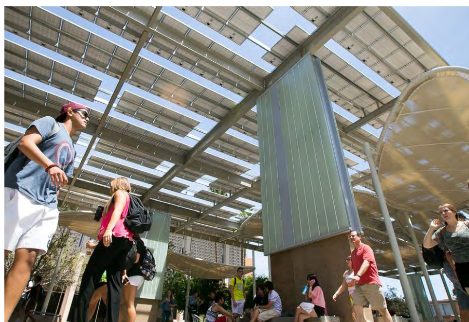
Solar panels create a canopy over public space outside Arizona State University's Memorial Union
