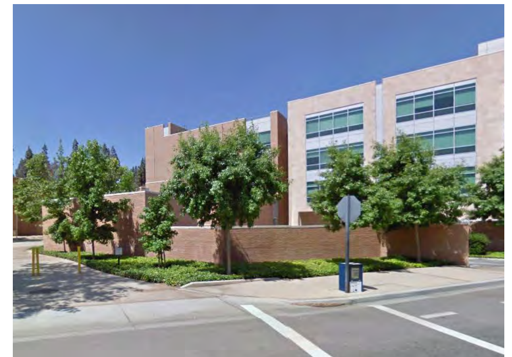
Brick wall screening service yard at Chung Hall, UC Riverside
