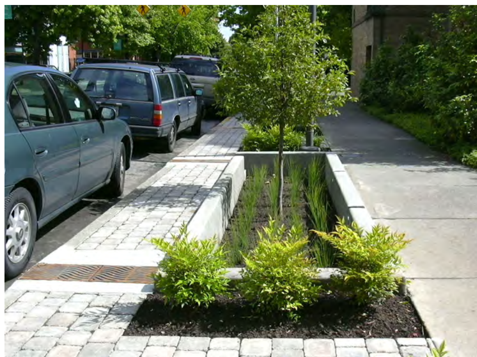
Stormwater planter integrated with sidewalk, Portland State University
