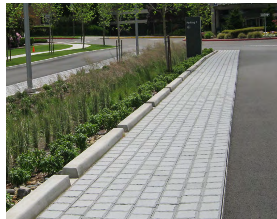
Example of stormwater swale integrated with street edge, Portland
