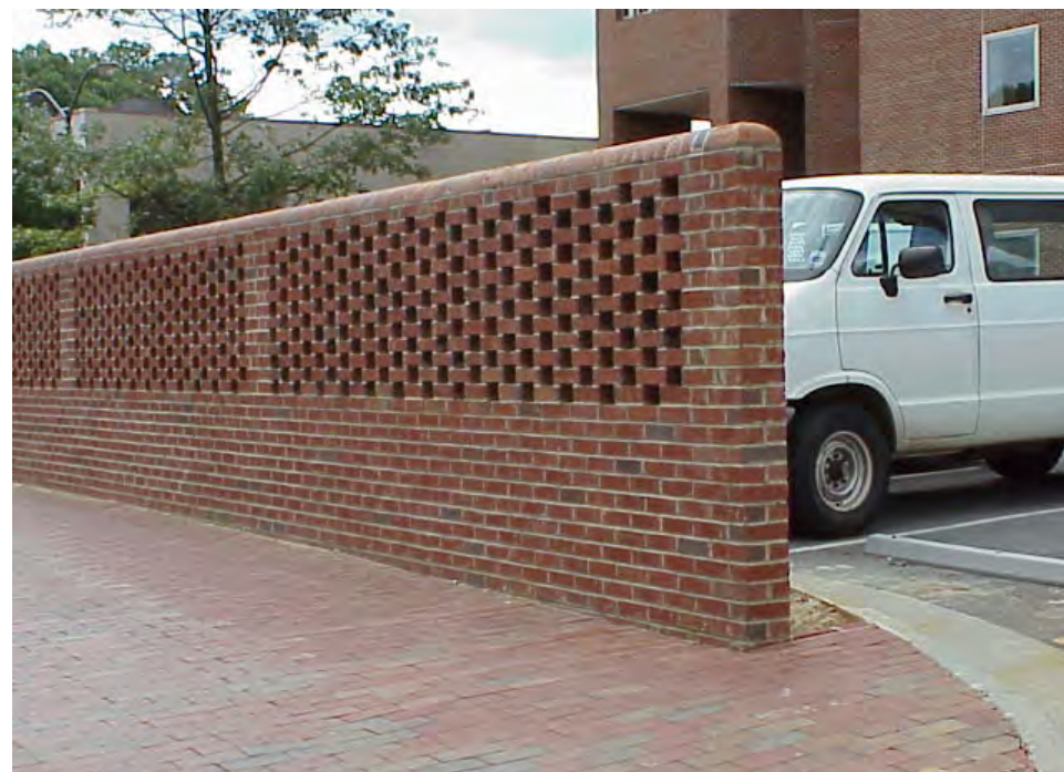
Brick screen wall, UC Davis
