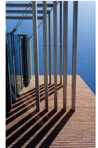
Shading at Exposed Fenestration
