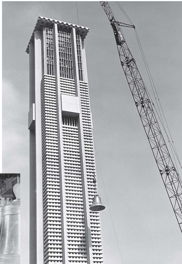
Construction of the Carillon Tower
