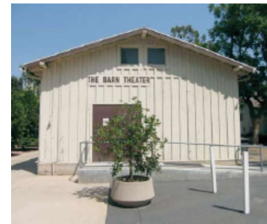
Barn Theater – West Façade
